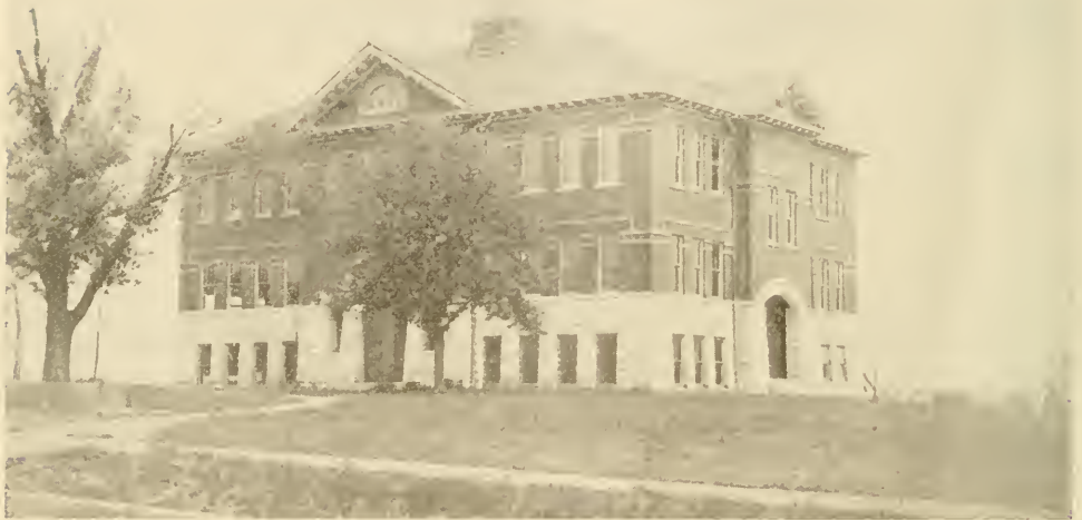
HIGH SCHOOL BUILDING, AUGUSTA, KANS.
