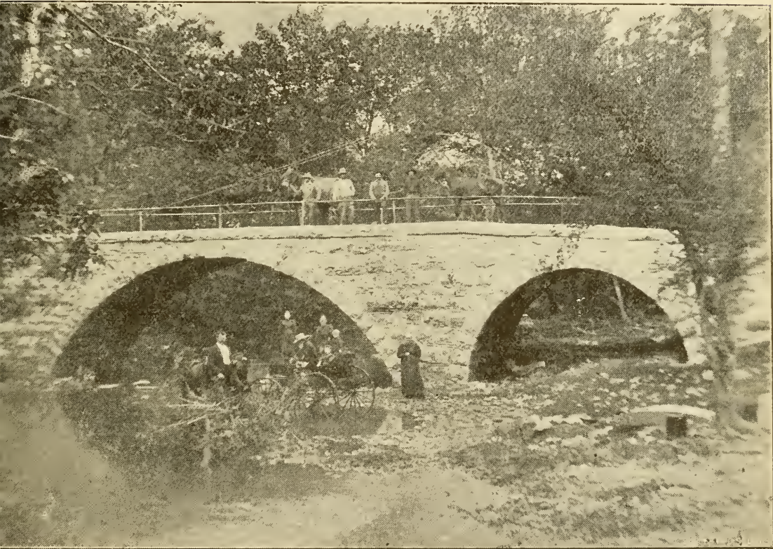
NORTH MAIN STREET BRIDGE, EL DORADO, KANS.
